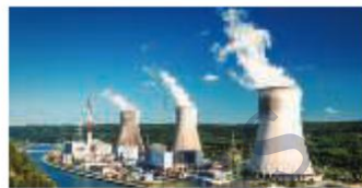
▲ Figure 14 This nuclear power station uses nuclear fuel to power a turbine. The cooling towers in this nuclear power station act to keep the temperature T_c as small as possible, so that the efficiency is improved.
