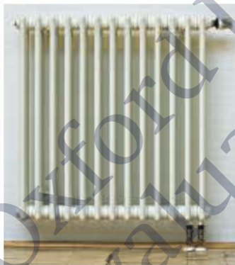
▲ Figure 22 A radiator, used circulate hot water to heat a room.
