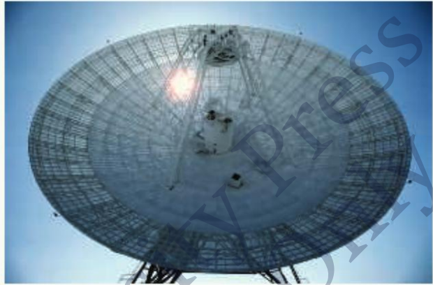
▲ Figure 13 Radio waves interact with matter very differently to visible light—as a result, the mirror on this radio telescope does not look like a mirror for visible light.
