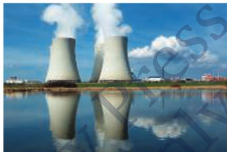
▲ Figure 5 A nuclear power station.
